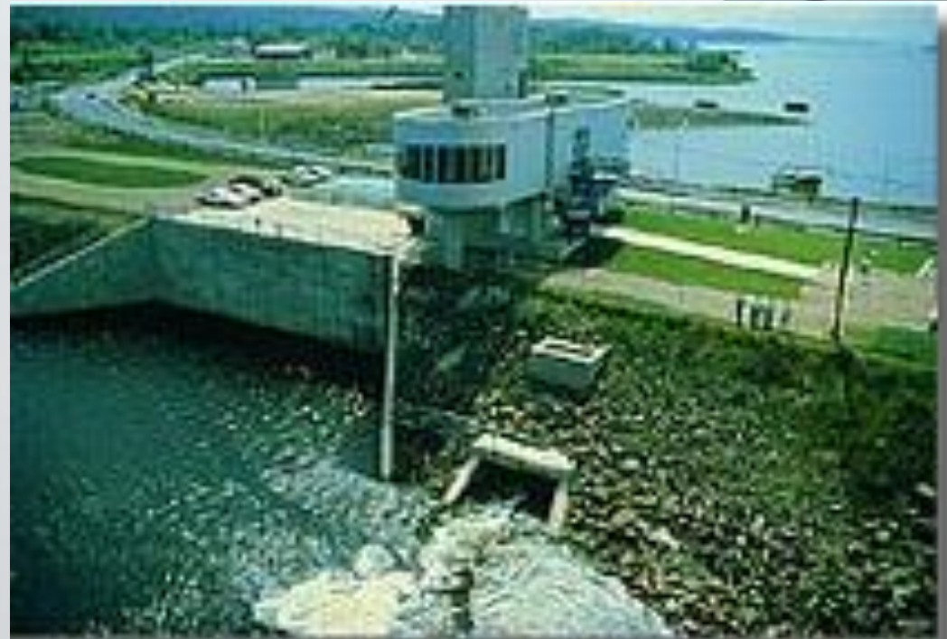
Tidal Power Plant in Annapolis, NS
