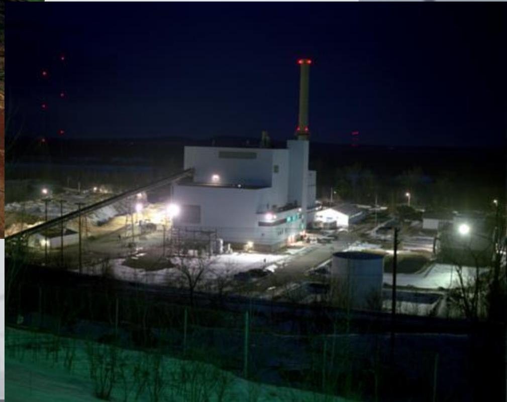
Biomass (Wood-Fire) Power Plant, USA
