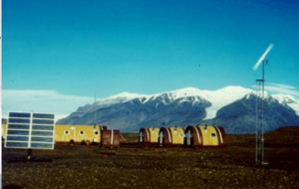
Photovoltaic array for a hybrid system at the Warden Station in Ellesmere Island National Park in the Canadian Arctic
